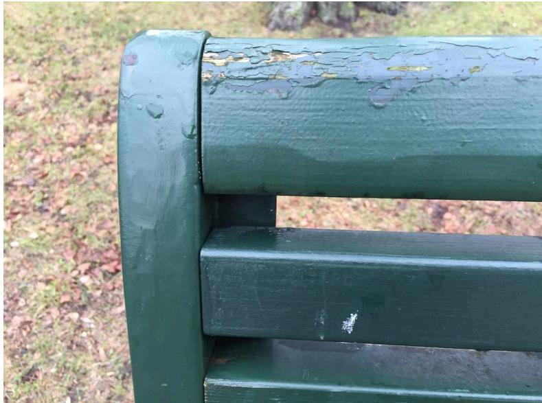
In parallel, **graffiti** posed a significant operational challenge. Painted wood absorbed both moisture and graffiti pigments, making cleaning difficult and often ineffective. Repeated graffiti removal accelerated surface wear, further shortening the service life of the benches and increasing labor intensity.
